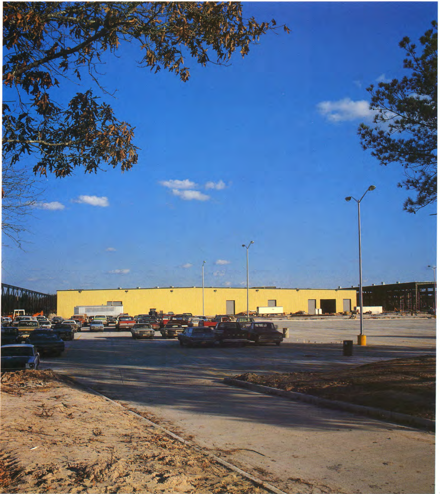
A new $7 million plant for structural fabrication, final assembly and shipping operations was built in 1981. Full production in this plant is scheduled for mid-1982.
