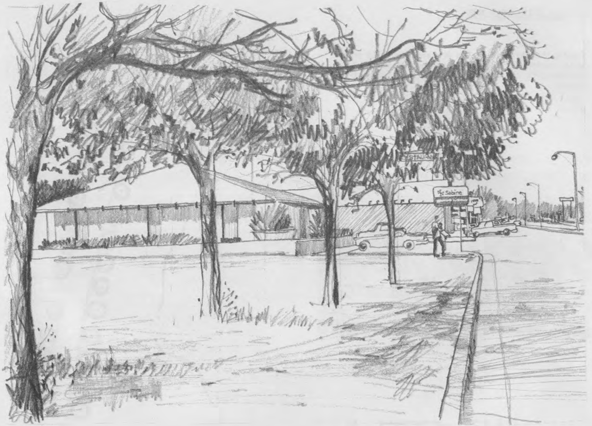
View of Sabine Development Company looking north from feeder road off U.S. 59.
