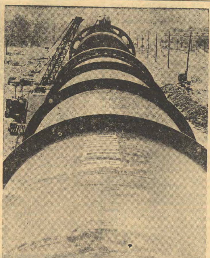
One of the world's largest single pieces of precision mechanized equipment, a 300-foot rotary kiln for the manufacture of cement, is being completed at the Texas Portland Cement Plant at Orange, Texas.
