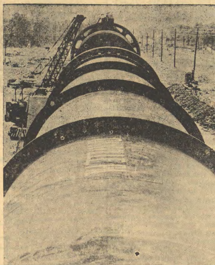
One of the world's largest single pieces of precision mechanized equipment, a 300-foot rotary kiln for the manufacture of cement, is being completed at the Texas Portland Cement Plant at Orange, Texas. The kiln will convert oyster shells into regular and special types of cement. Those responsible for engineering and constructing the facility have designated it as 'the world's most modern cement plant'.
