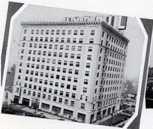
Petroleum Securities Building. Headquarters of the Petroleum Securities, Pacific Western and several Independent Companies.
