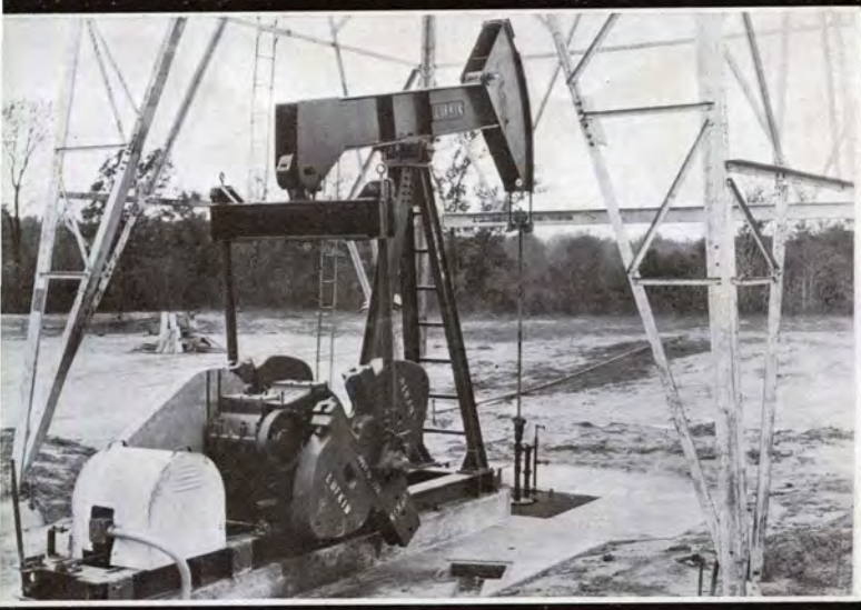
Stanolind Oil & Gas Co., Wooley Lease, Hooper Survey, East Texas — LUFKIN Unit Assembly T.C. No. 3-22 with long base for electric motor drive.
