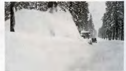
Heaving snow with an Augur type rotary plow on the Susanville lateral of California.
