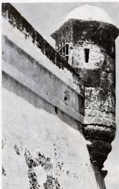
One of the 27 Bastions and part of the historic wall surrounding Cartagena. It is 40 feet wide in places and many sections are in such good repair that a car may be driven along the top of the wall.—Photo courtesy United Fruit Co.
