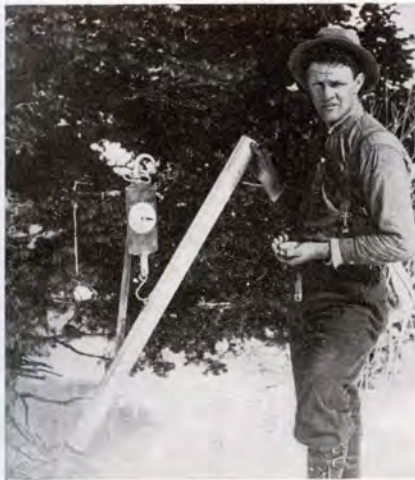
The snow surveyor determines moisture content of snow by filling the tube shown and weighing it. Moisture content is a guide to the heaviness of the job of snow removal and sometimes dictates types of machine equipment to be used.
