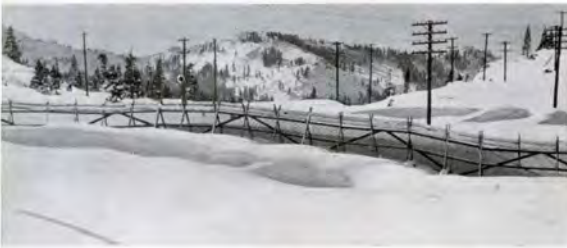
Though the snow here shown at The Donner is mild, the use of drift fence is shown. It forces snow to drift at a point off the highway, easing the work of the snow removal forces. It is interesting to know that much of this snow fence is manufactured in the "Sunny South" and particularly in LUFKIN, TEXAS.
