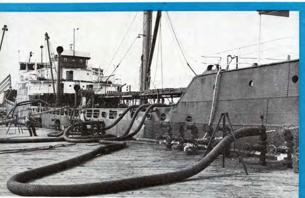
Loading modern oil tanker in Los Angeles Harbor.
