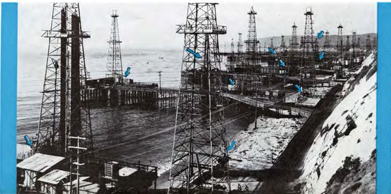
Elwood field, Goleta, California—Mountainside view looking into the Pacific Ocean. Arrows point to Lufkin installations. There are thirty to forty Lufkin Units not visible in this photograph.
