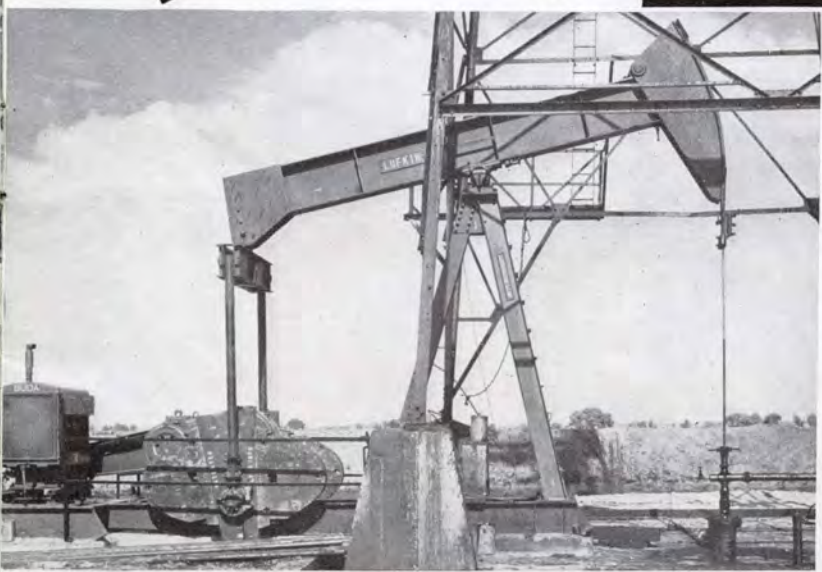
Shell Oil Company, Mountain View, Lufkin, T.C. 1-41 unit assembly.
