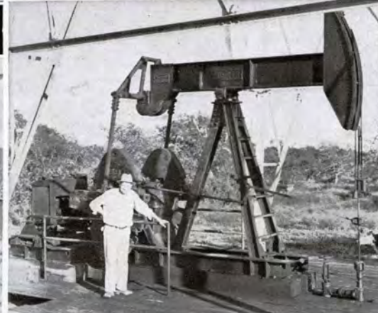
Lufkin T.C. 3-22 Unit installation for major oil company in the Dirks field, Bee County, E. D. Miller, Pumper.
