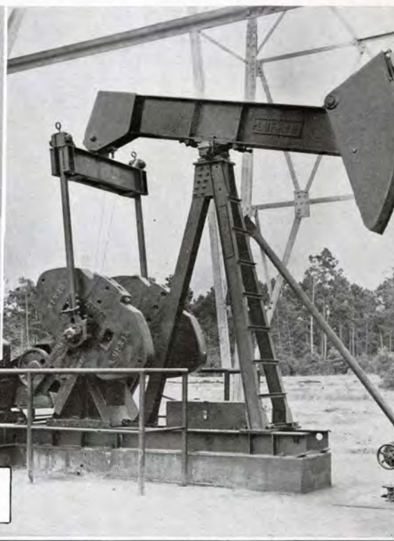
Major oil company installation of Lufkin T.C. 3-22 Unit in the Conroe, Texas, field.
