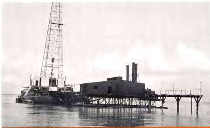
Marine operations along the Louisiana Coast have greatly increased oil production in several areas. This picture shows one of the major oil company's drilling and boiler barges that float or sink, as the occasion demands.
