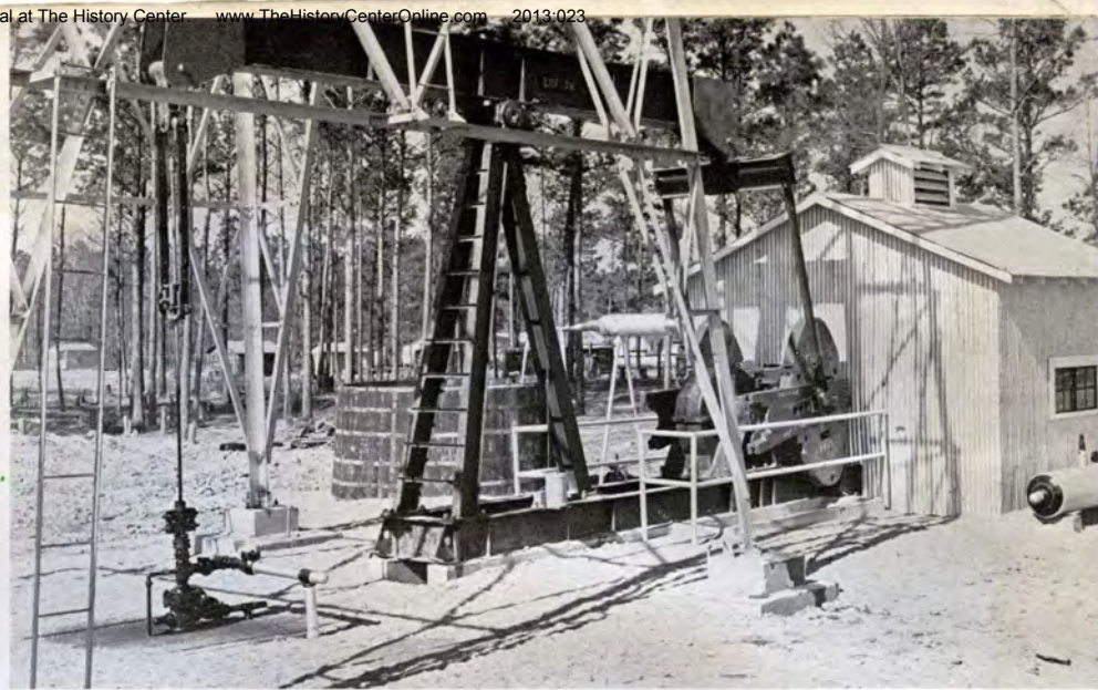
Lufkin T.C.-54 Unit on 6000 ft. well for major producer in Rodessa field.
