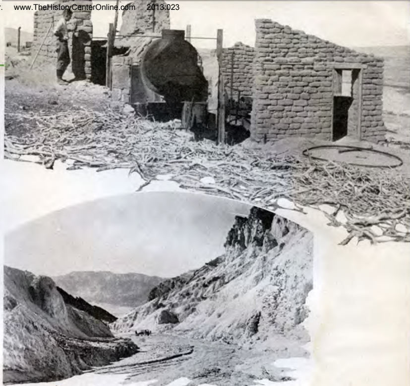
Top: Back in the early '90's this ruin was the one big industrial activity in Death Valley. The first refined borax produced in the United States came from this spot, called the "Harmony Borax Works." The sticks in the foreground are mesquite roots, used as fuel in the old boiler shown. The ruin is one of the tourist attractions of Death Valley.
