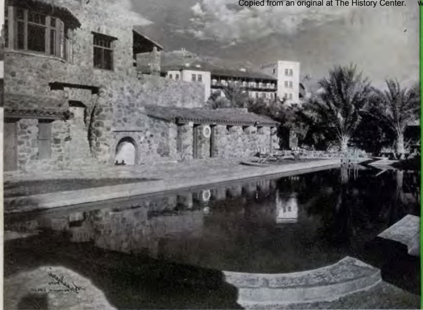
Swimming pool and north wing of Furnace Creek Inn.
