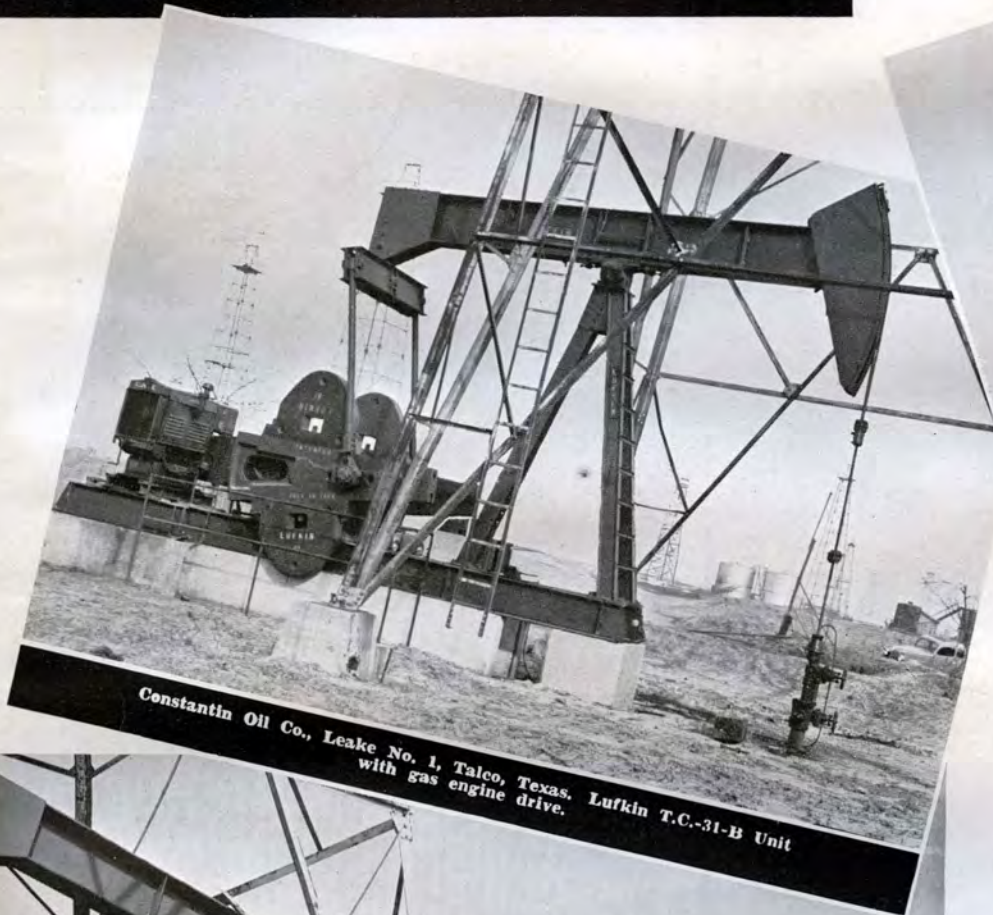
Typical Lufkin installation in the Talco, Texas, field. Magnolia Petroleum Co., W. H. Crawford No. 1, Lufkin T.C.-58 Unit with long base.
