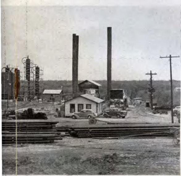
Refinery Co., now under construction and operation about March 15.
