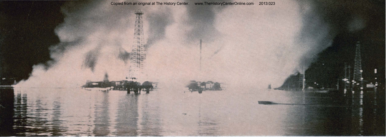
CLOSE-UP OF FIRE FROM SEA WALL.
