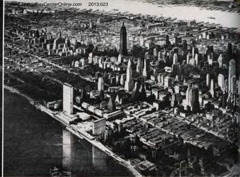
THIS BIRDSEYE view of the United Nations permanent home on the East River site shows it in relation to the central area of Manhattan.
