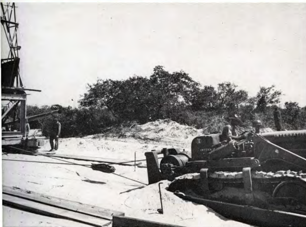
IN FIVE HOURS , this standard drilling rig with machinery on the floor was moved to a new location of one-half mile distance by a Model 60 on a TD18 Tractor. Approximate weight was 260,000 pounds.
