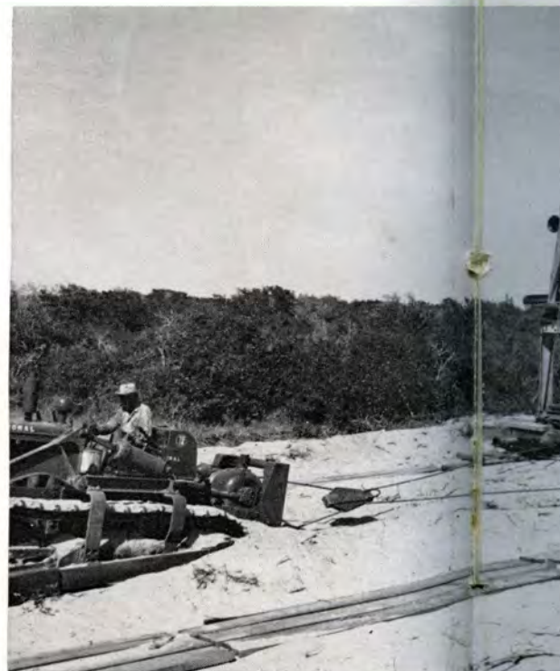
IN FIVE HOURS , this standard drilling rig with machinery on the floor was moved to a new location of one-half mile distance by a Model 60 on a TD18 Tractor. Approximate weight was 260,000 pounds.
