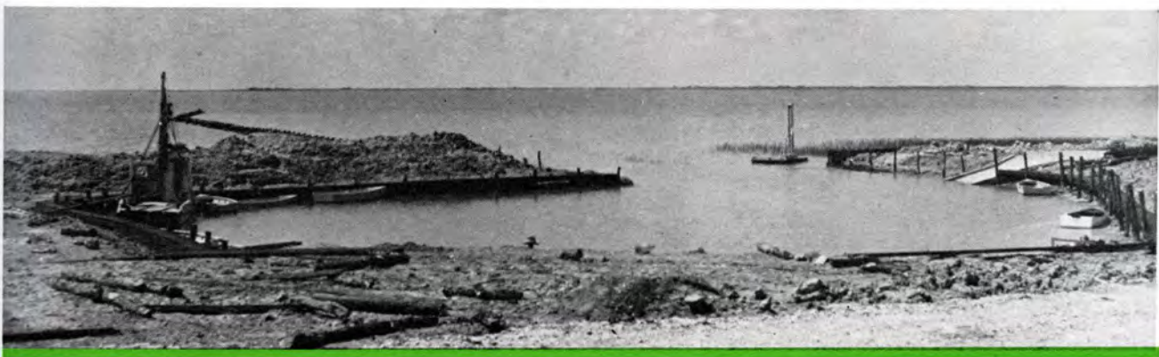
This recently completed boat basin provides a safe harbor when the weather gets rough.
