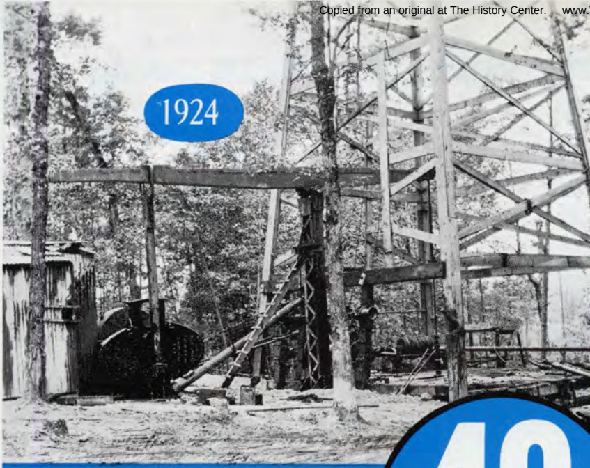
THE FIRST LUFKIN PUMPING UNIT WITH TROUT COUNTERBALANCED CRANK ILLUSTRATING THE ORIGINAL DESIGN.
