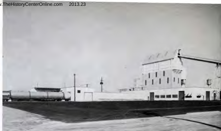
CROWE-GULDE Cement Company, organized 39 years ago, built a new completely automated block plant in 1961
