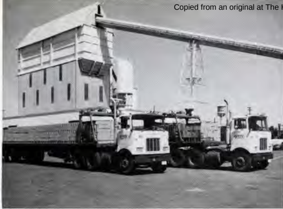
LUFKIN HTS trailers haul Crowe-Gulde's products throughout the 250-mile radius of Amarillo which they serve
