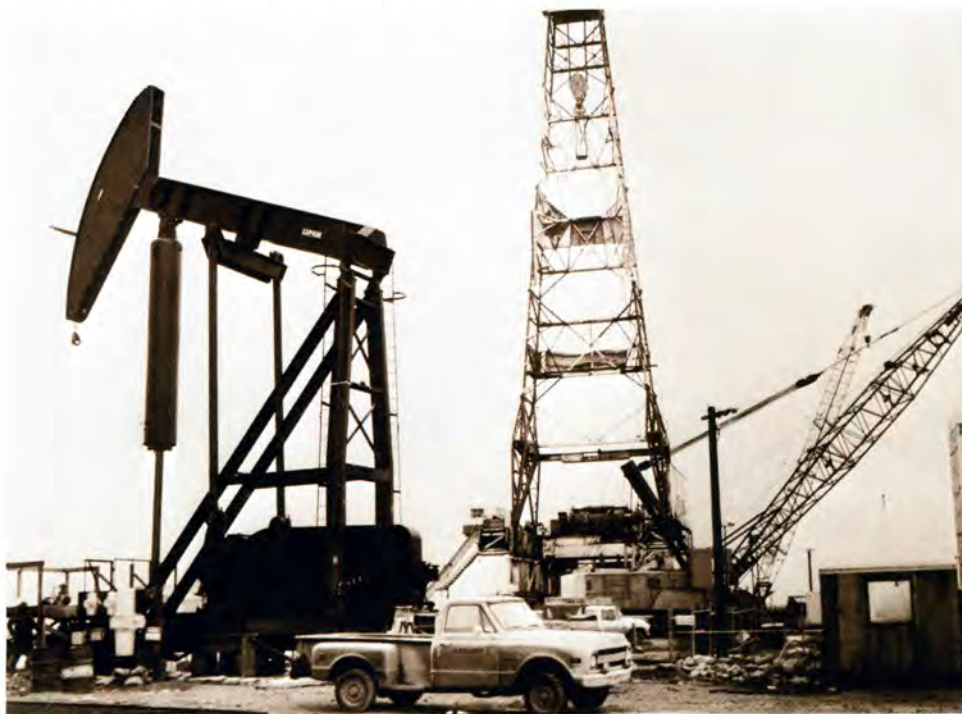
At left is the LUFKIN Air Balanced pumping unit on location at the Atomic Energy Commission's recent "Cannikin" nuclear underground test on Amchitka Island, Alaska. The rig in the background was used to drill the access shaft leading to the detonation cavity.
