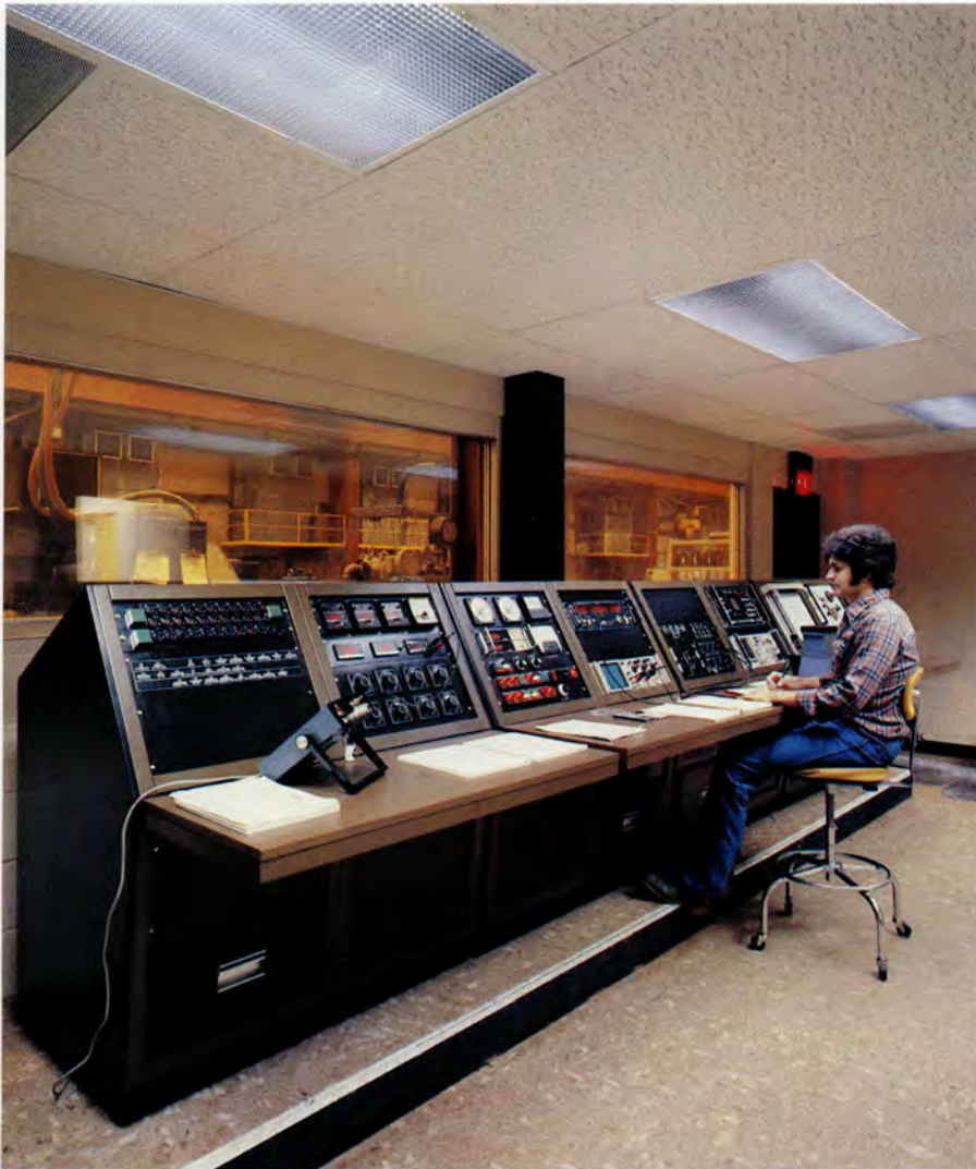
(Opposite page) The new testing facility for enclosed gearing was part of the recent gear expansion at Lufkin Industries. It features testing areas for both high-speed and low-speed precision gearing. (Above) The test panel was designed to provide data display, data recording, control of test parameters and instrumentation for diagnostics of gear quality problems. Pictured is technician Clarence Miller.
