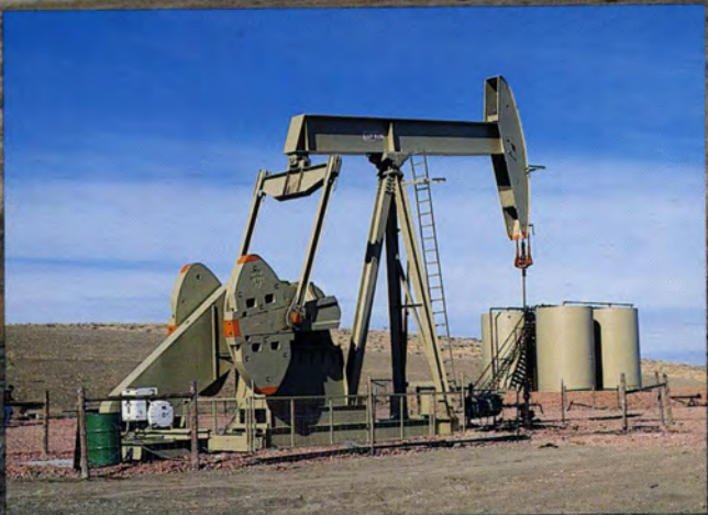
LUFKIN C-912D-365-168 Unit, Puma Petroleum Company, Campbell County, Wyoming.
