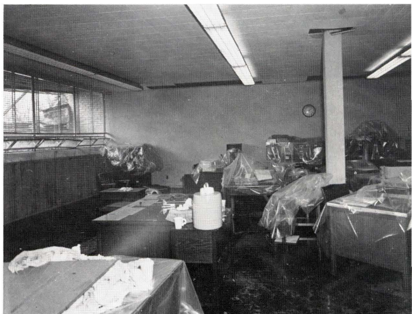
A CONCRETE floor in the Engineering department located directly above the Accounting department shown here saved this office from fire, but heavy water and smoke damage was suffered
