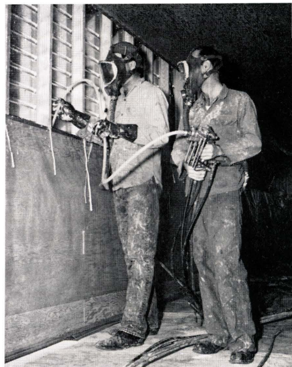
TEER and EIRBY McADAMS are foaming the first four feet of the sides of a trailer
