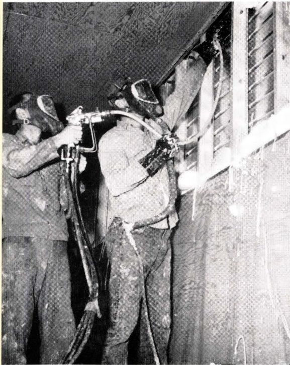
AFTER the walls have been foamed to six feet, the ceiling of non-meat rail trailers are foamed before the other four feet of the sides are completed. Here TEER and McADAMS are putting the gun in the ceiling to start foaming
