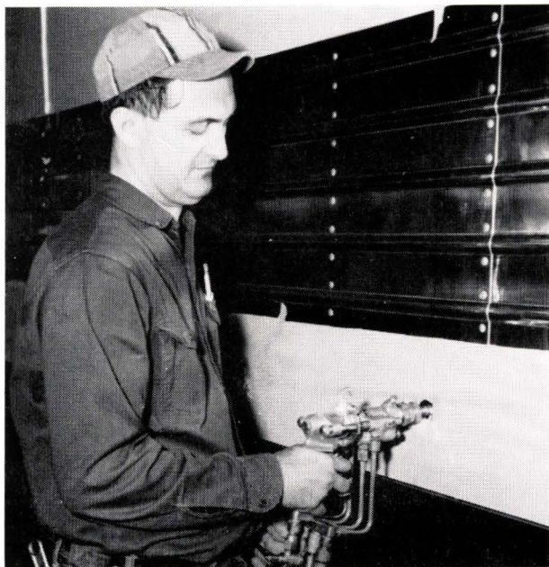
LUM GENERAL TEER puts 8-foot tube in hole outside of trailer to begin foaming the floor. Floor fills are on 24-inch centers
