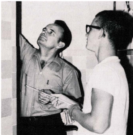
CHARLIE and his son are hanging the shower rod as the last thing to be done to the new bathroom Charlie built
