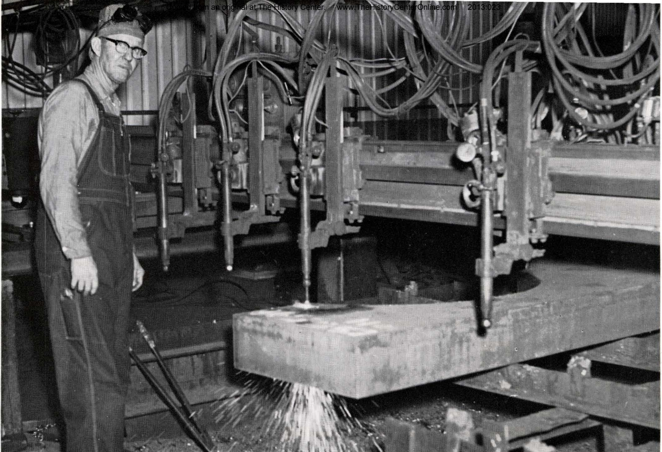
1. IN THE WELDING and Structural Shop, the first step is burning angles and curves into plates of rolled steel with the shape burner's torch, an automatic burner controlled by an electronic eye which follows the desired pattern on a penciled drawing. Operator is J. D. Edwards, first shift.
