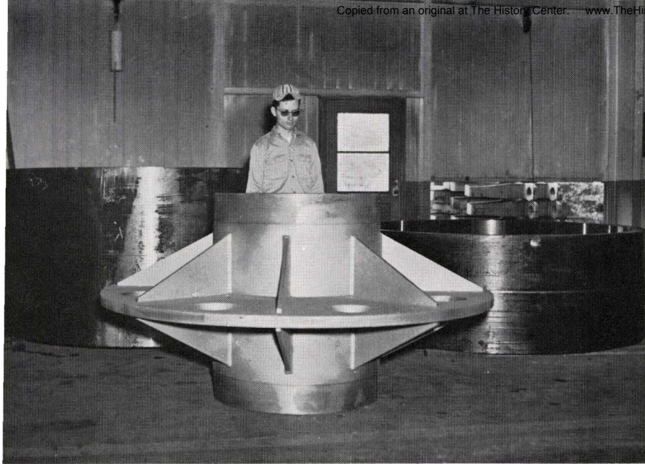
3. MEANWHILE, the procedure is underway of welding the gear "blank," the name for a gear without the teeth cut. Here the spherical "hub" has been welded to the "webs," round discs which, when welded inside the gear blank's outer rim, will provide internal stress for strength. Pictured is Ronnie Hunt, Welding Shop, first shift.
