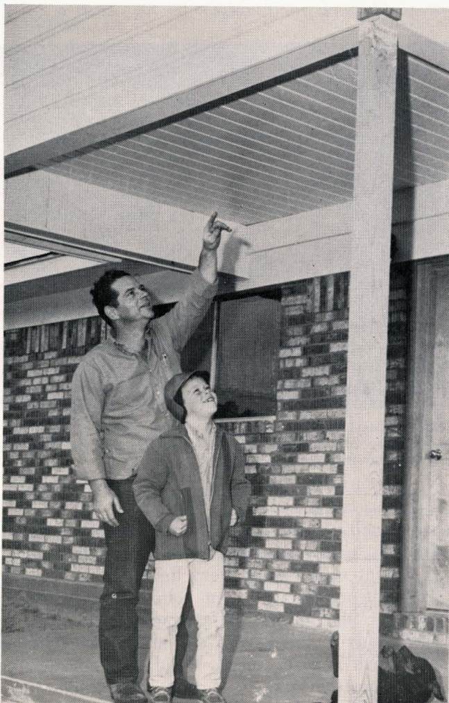
WHITE trim and turned wooden posts will complete the exterior's colonial styling. Dan and Danny examine the temporary brace soon to be replaced by posts
