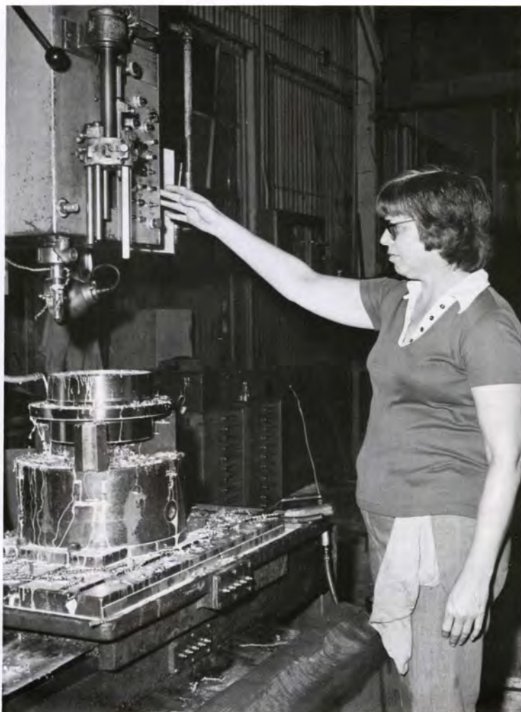
Right: Dora May Hight is training on a 244 drill press which positions, drills and taps parts as instructed by the computer tape which runs its cycles
