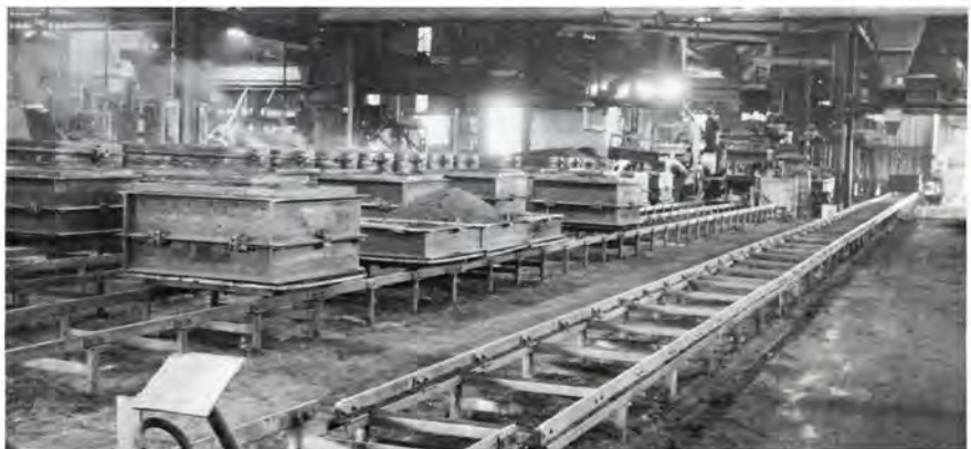
Conveyors in the "green" sand molding bay
