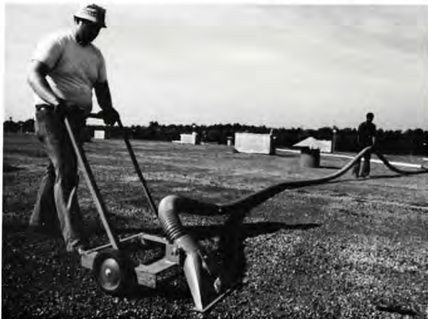
A crew from Michigan vacuumed the rock covering off trailer roof
