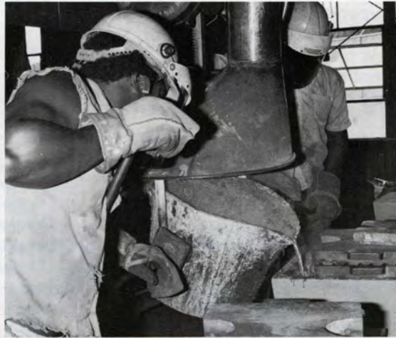
(Left) Don Price, aluminum and brass foundry, 1st shift, pushes completed mold made on pep set to assembly line to be poured. (Above) Calvin Jones, aluminum and brass foundry, 1st shift, charges the furnace with brass shavings. (Below left) Don Price, left, and Michael Hulett, both aluminum and brass foundry, 1st shift, bringing the ladle of metal to pouring line. (Below right, upper) Bronze bushing being poured. (Below right, lower) Foundry personnel built table to shake castings out of molds
