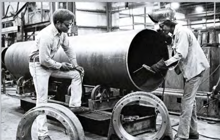
(l-r) Therman Davis and Clarence Owen with automatic tank roller
