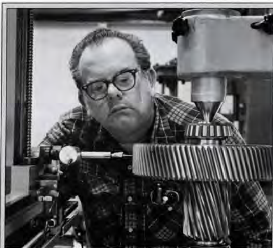
Helping to control quality, Jerry Tullos, gear specialist inspector, checks the spacing between gear teeth. Photo by Viron Barbay
