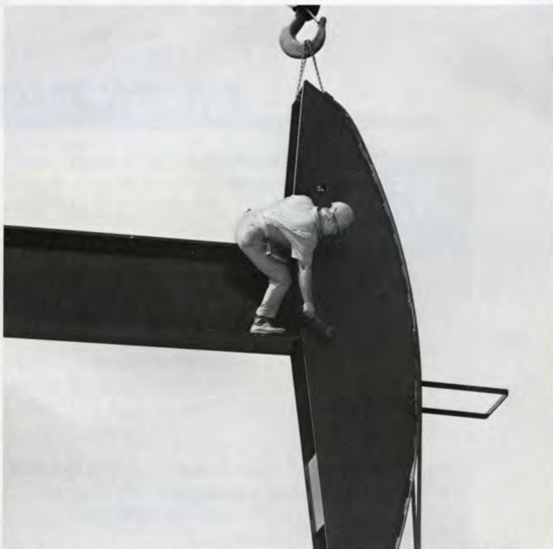
Left: W.Z. Hutson (top), John Bridges (middle), and T.J. Reynolds (bottom), guide a counterweight into position for mounting on one of the C1280 cranks.
