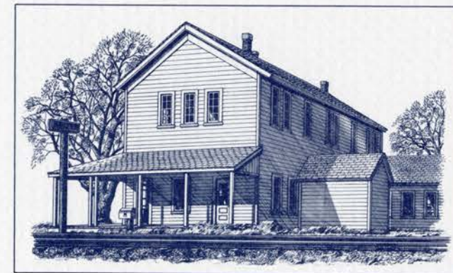
The Angelina and Neches River Railroad, which was chartered by the state in 1900, operated from this two-story building at Keltys for many years. The structure, built in the late 1800's, also served as the main offices for Angelina County Lumber Company before the firm built its own offices at Keltys. The building was demolished in the 1950's.
