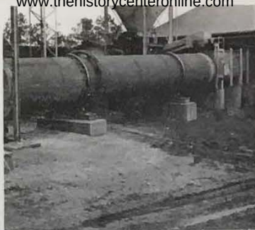
Huge, diesel heated drier can turn out 15 tons of clay or 7½ tons of lignite coal per hour.
