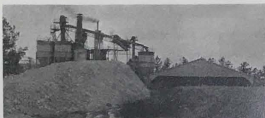
Stockpiles of East Texas bentonite (left) and filter clay (right) are draglined into building (rear), run through grinder, then fed into drier.
