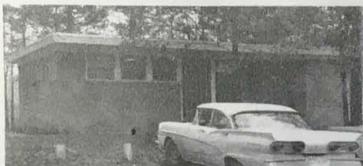
Zavalla plant office sits among the pines and oaks some 100 yards from production building.
