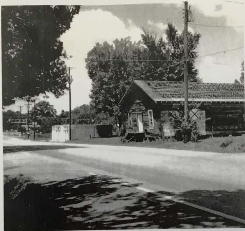
BARGE FEED HOUSE being torn down in 1992
